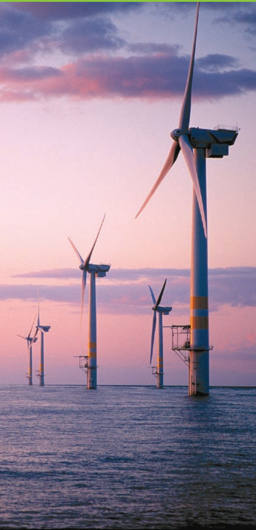
To ensure continued industry growth, DOE's Wind Program is conducting research in new applications such as offshore developments like the Arklow Bank Offshore Wind Park. Located about 10 kilometers off the coast of Arklow, Ireland, the park consists of seven GE Energy 3.6-MW wind turbines.
